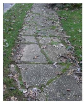
The seller reported the driveway to be 4 years old. This relatively new driveway contains multiple cracks. We believe the cracks are due to a nearby tree spreading its roots under the driveway. It is recommended that the trees growing near the driveway be removed. Also, the cesspools are located under the driveway. It is strongly recommended that the cesspools be inspected prior to closing for possible damage.
