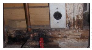
Please note, this is the only visible sill plate in the basement (or the slab section of the house) and this location contains termite damage. There is a very good chance there is other termite damage to the hidden wood framing. Make sure the sellers has the property treated for termites and obtains a transferable and renewable guarantee.
